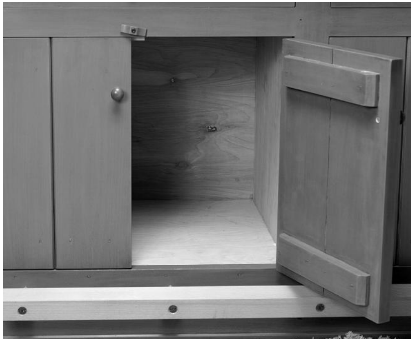
Board and batten door.
