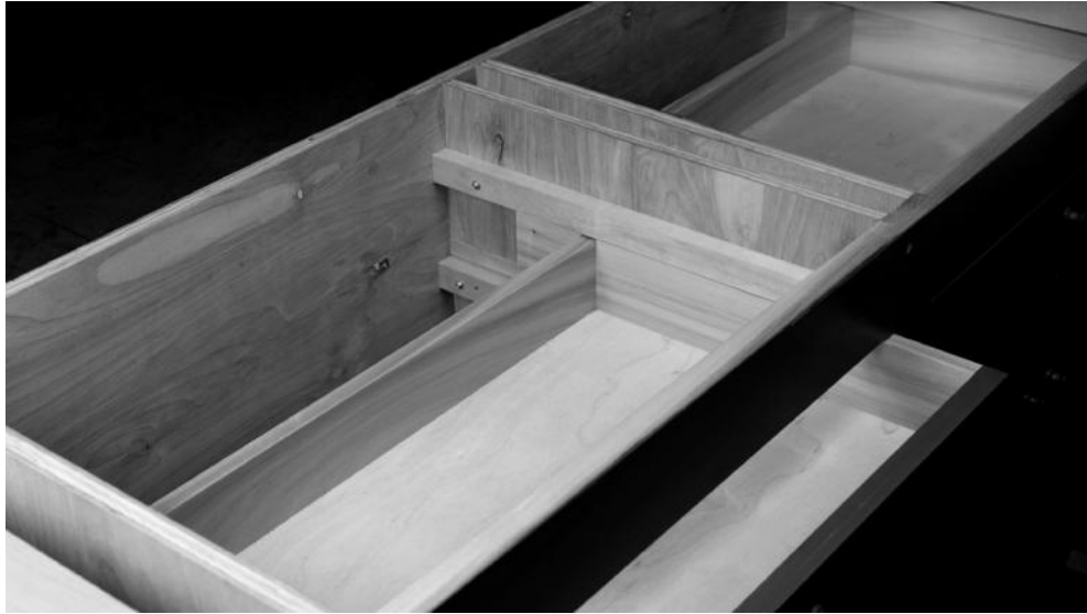
Drawer and runners showing adjustable screws in the runners.
